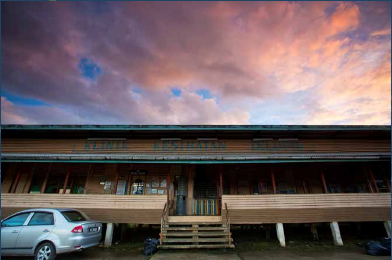
Frontal view of Primary Health Clinic at Telupid, with a back drop of setting Sun showing its hues.
